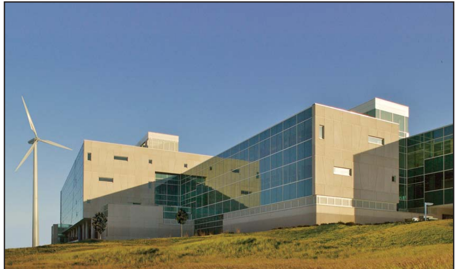
The new headquarters of Great River Energy, your electric cooperative's wholesale power supplier, is one of the most energy-efficient buildings in the country.
