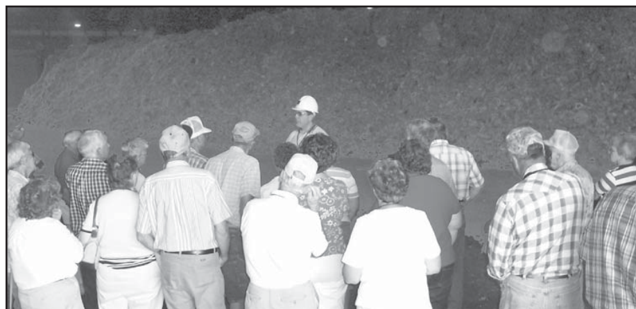
Mountains of shredded garbage become fuel to create electricity at Great River Energy's Elk River power plant. Co-op members also toured a peaking power plant and a wind turbine.
